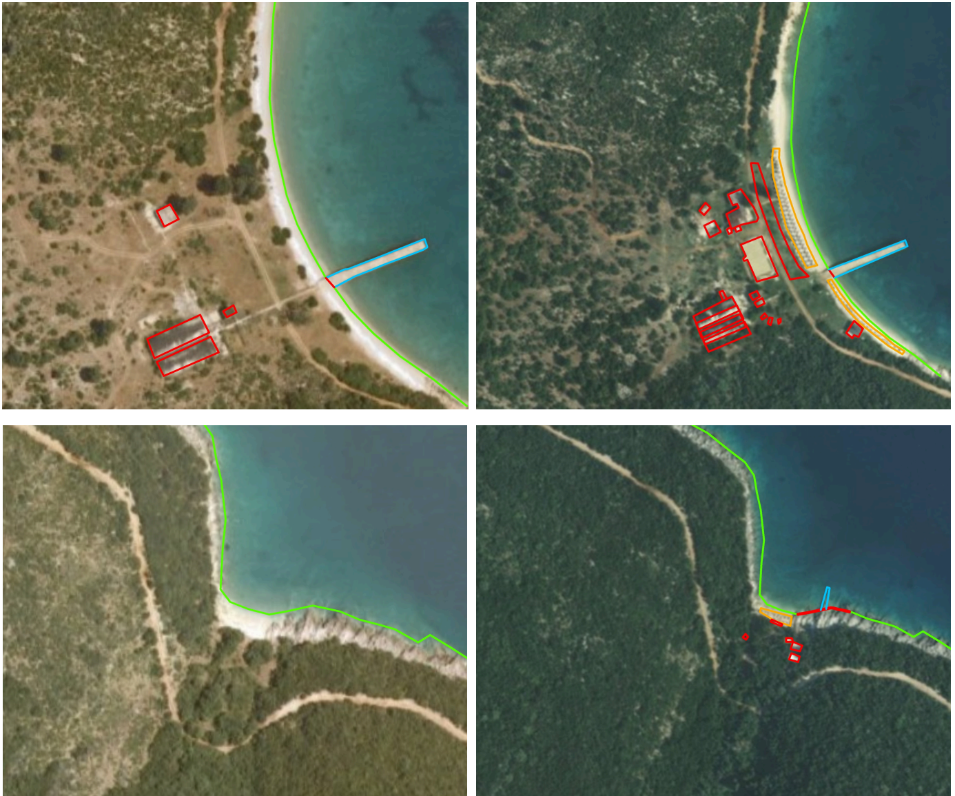
Figure 27. Changes in the infrastructure of the beaches of Karaburun-Sazan MPA from 2007 (left) to 2022 (right). Shen Vasil in the first photos and Dhimkushta in the second photos.
